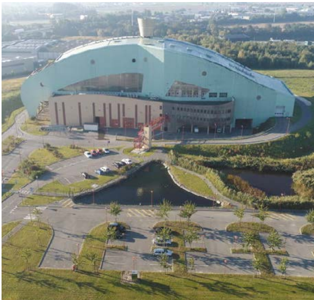
Flamoval energy recovery center
