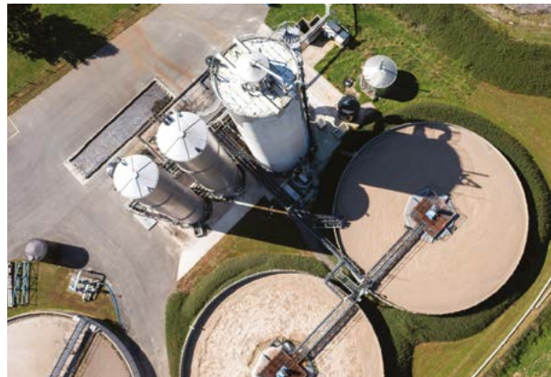
Cartonnerie Gondardennes wastewater treatment plant
